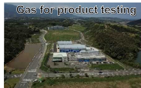
Hydrogen Energy Test and Research Center (HyTReC)
